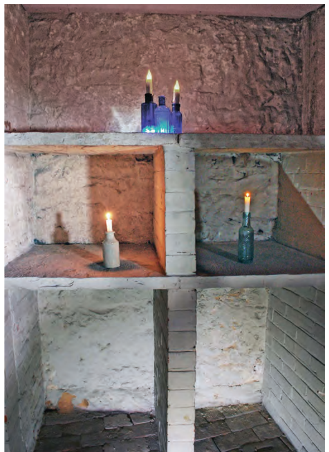
Brick-built storage bays which are very similar to those at the White Horse inn
